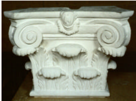
Repaired with plaster
